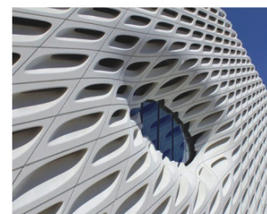
Tilt-up panel system / GRC panel
